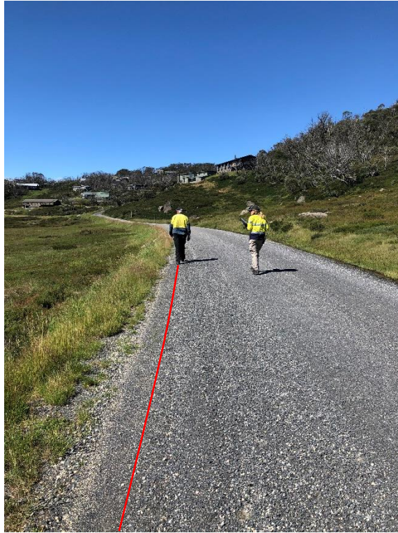
Image 3 - looking south along Perisher Creek Road. Red line indicates approximate location of trench for water, power and communications to hydrant 2.
